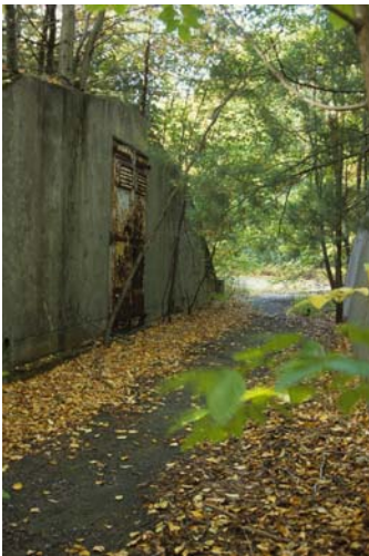
NAD Hingham Annex - 1989
